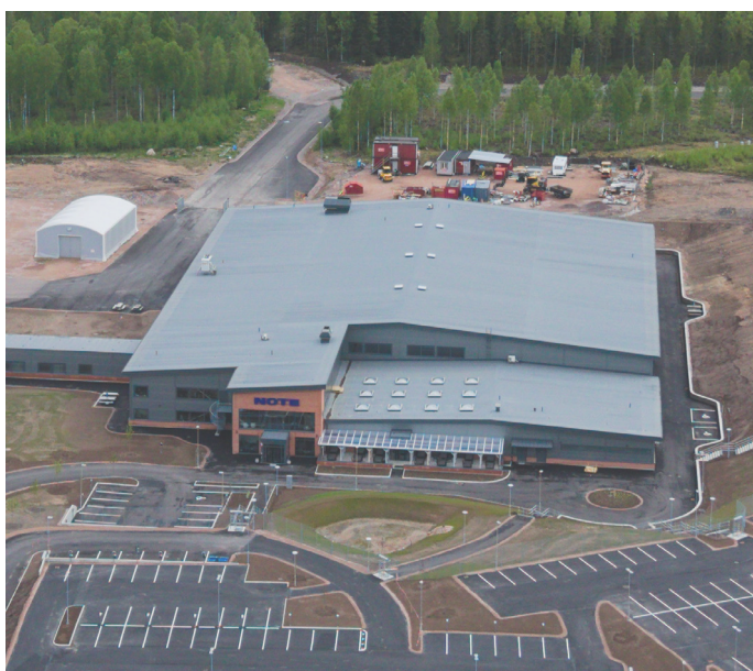
NOTE's new state-of-the-art plant in Torsby, Sweden, which adds about another 7,000 m 2 of production area.
