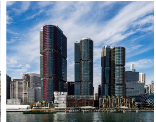
International Towers, Sydney
