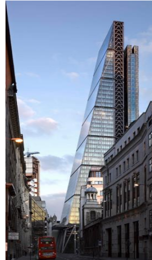
Leadenhall Building, London
