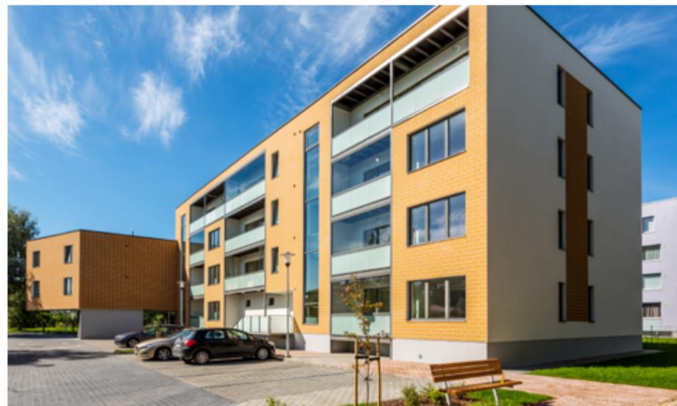
THE RÄÄGU 9 APARTMENT BUILDING IN TALLINN HAS A CATEGORY A ENERGY LABEL. COMPARED TO APARTMENT BUILDINGS COMPLETED IN THE PAST, THIS ONE HAS THICKER INSULATION IN THE EXTERIOR WALLS AND ROOF, ALSO TRIPLE PANE WINDOWS.
