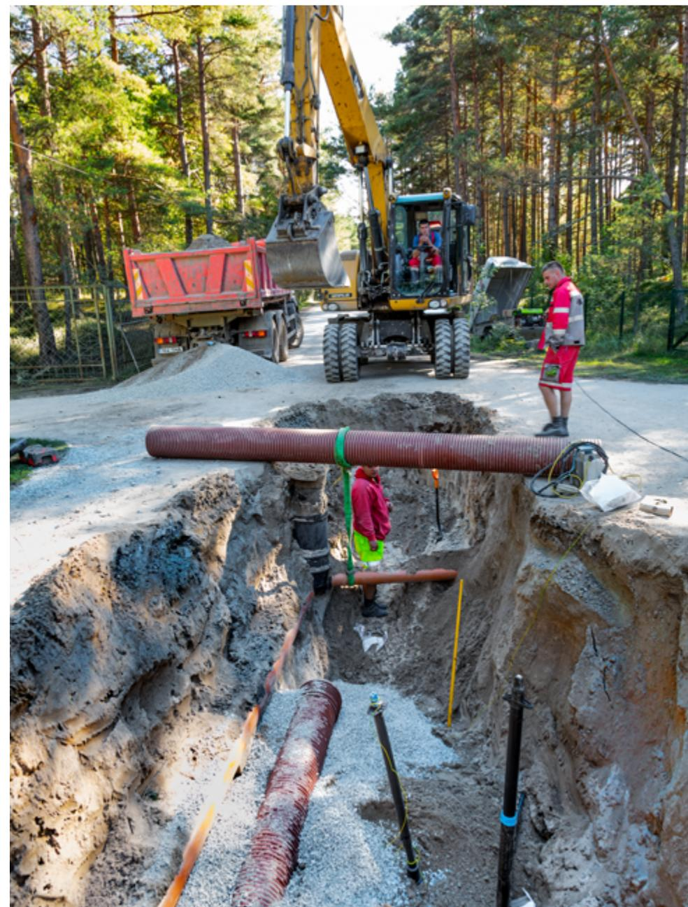
AT THE CONSTRUCTION OF THE VÄÄNA-JÕESUU WATER SUPPLY AND SEWERAGE SYSTEM, OVER 20 KM OF PIPE WAS LAID PER MONTH AT PEAK INTERVALS.
