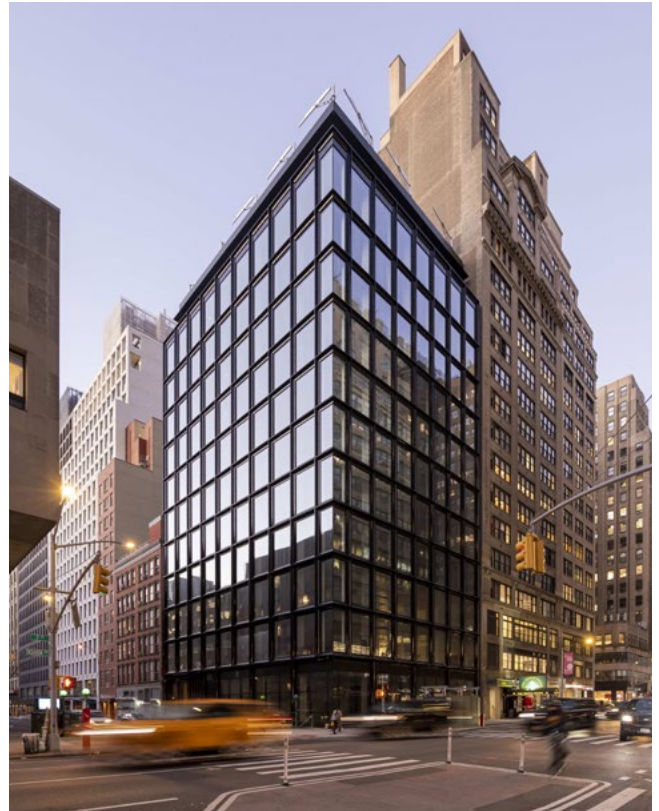
28&7, New York Corem's second largest ongoing project is a 12-storey office building at 28th Street and 7th Avenue on Manhattan.
